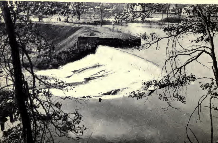
KNIFE SHOP DAM, SOUTH MERIDEN
